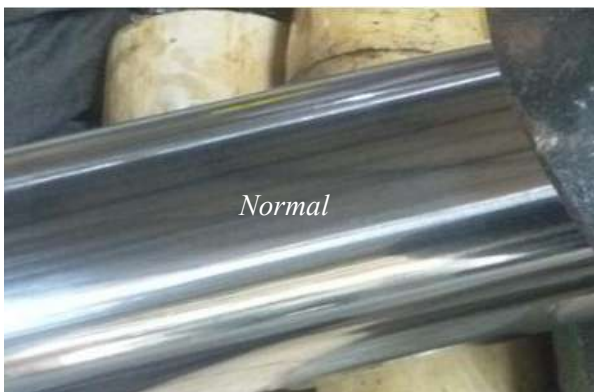
Fig. 6. Damage inspection of the cylinder rod condition in (a) experiencing wear on the surface, (b) experiencing corrosion, pitting, and peeling chrome layer, (c) normal condition or there is no wear, corrosion, and scratch on the surface.
