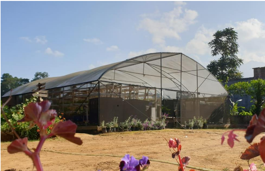
Aquaponics System Greenhouse
