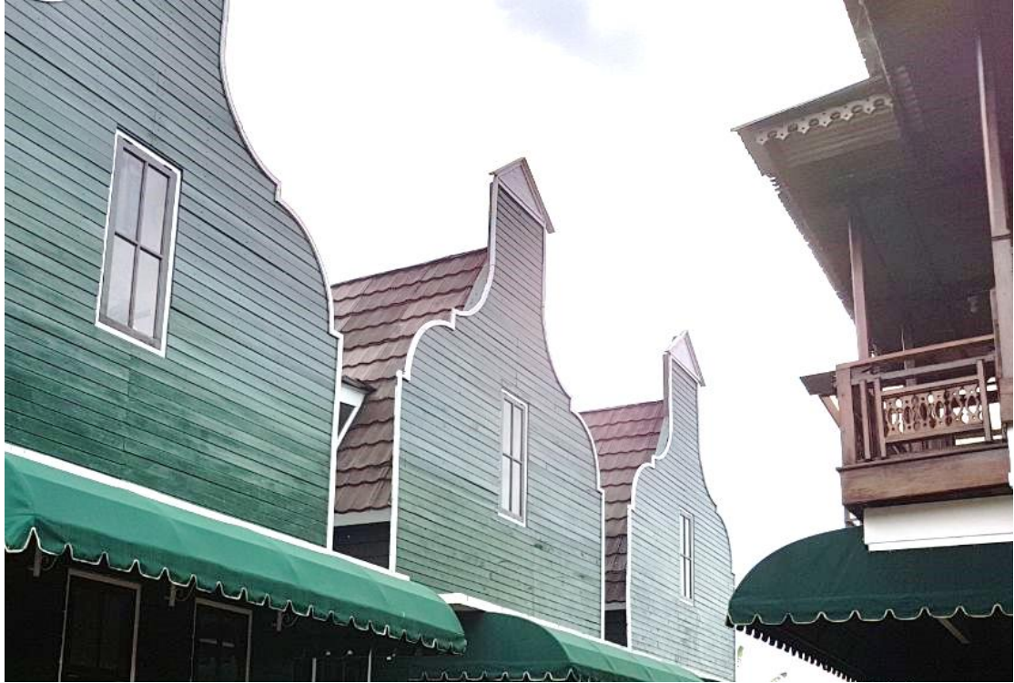
3 Units of Cottages for as one of Workshop and Training Facilities
