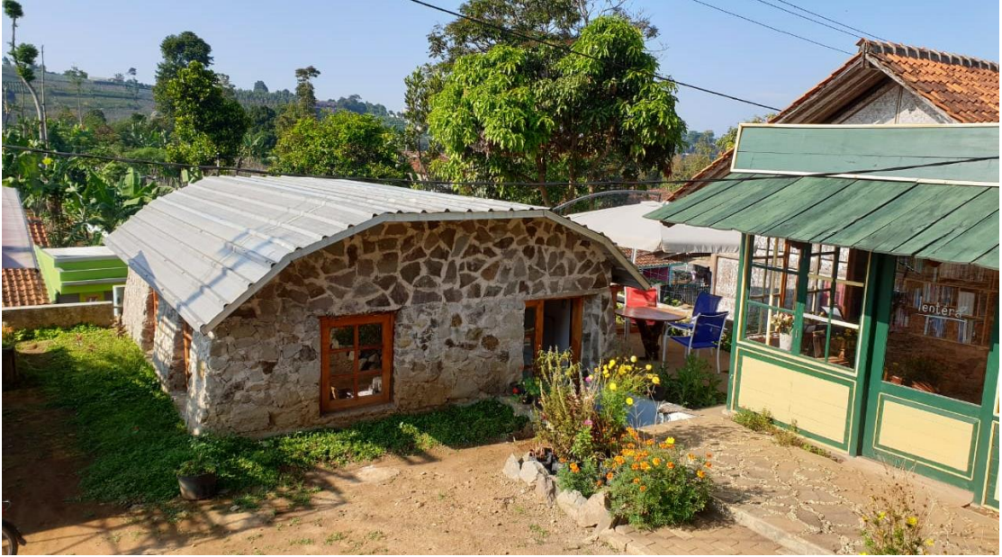
Processing Laboratory and office
